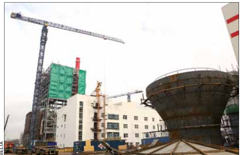
Construction site of plant in Svetlogorsk
