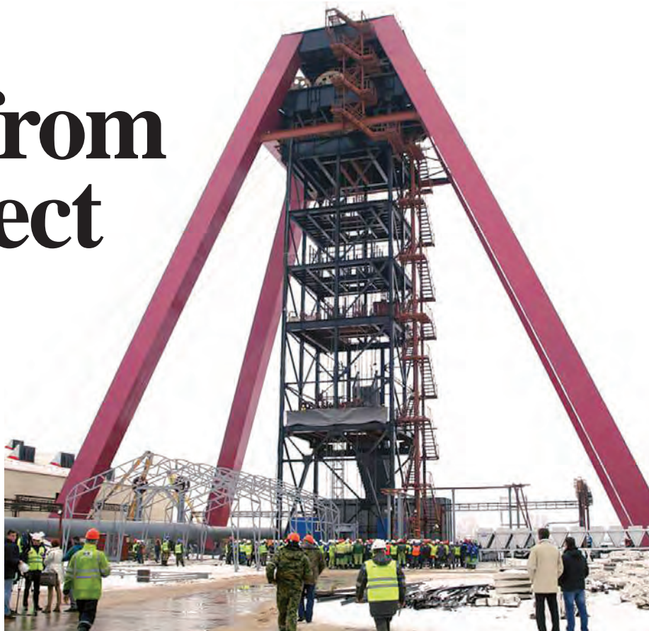
Construction site at Nezhinsky potash mining and processing factory
