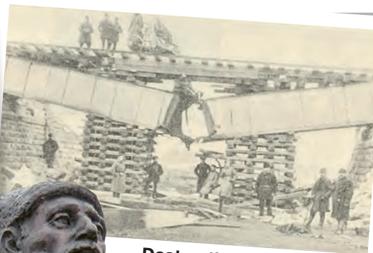
Destruction of the railway track near Wilno
