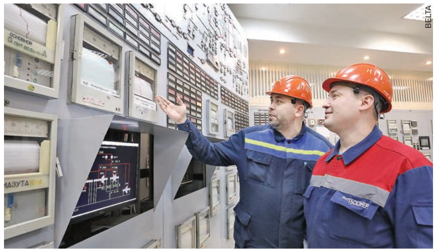
At Lukoml district power plant — the largest in Belarus
