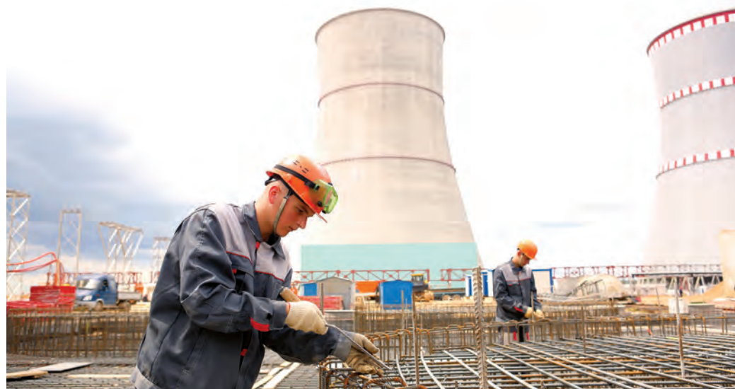
Installation works at the construction site of Belarusian NPP
