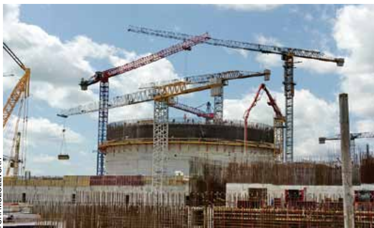
Assembly works at first power unit
