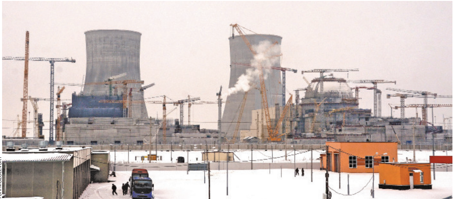
View on the construction site of BelNPP in Ostrovets
