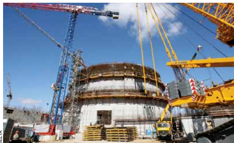
On the construction site of the Belarusian nuclear power station
