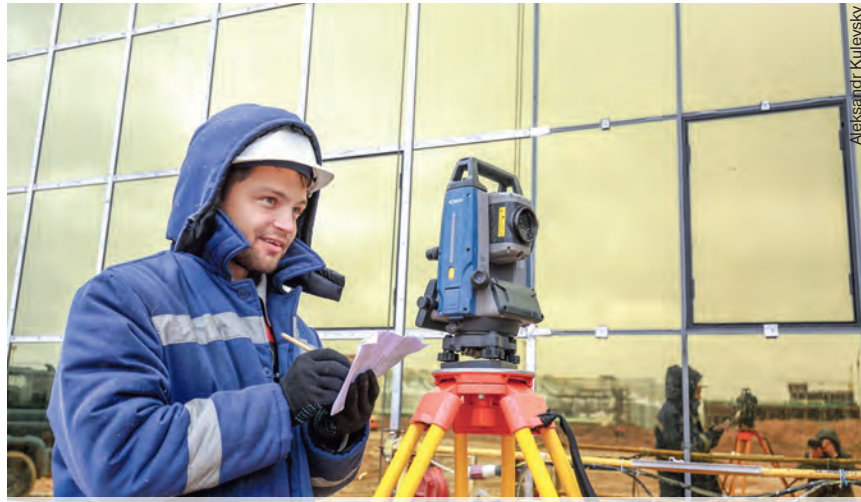
Surveyor Dmitry Prokhorchik at BNBC construction site
