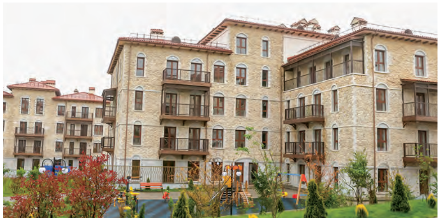
During a visit to Azerbaijani territories under restoration
