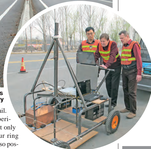
Equipment placed on a wheeled cart to be consistently moved along for about 150 metres
