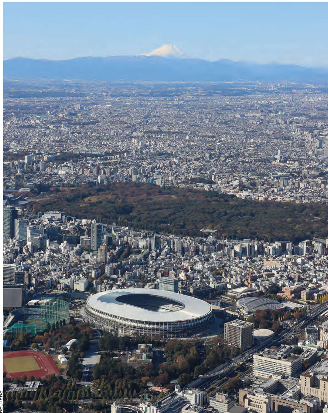
New National Stadium for Tokyo Olympics
