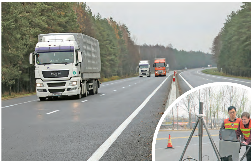
New method makes it possible to assess the roadway remotely without damaging its integrity
