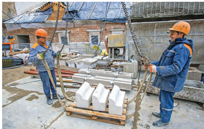
Work is in full swing at the construction site
