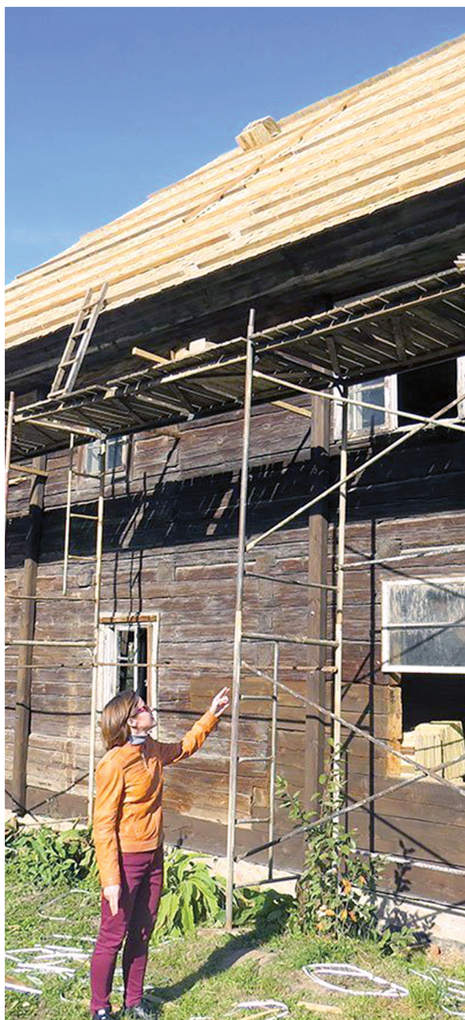
Reconstruction is underway
