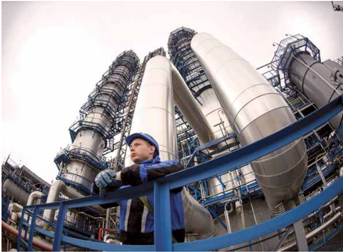
Modernisation at Mozyr Oil Refinery attracts the attention of investors
