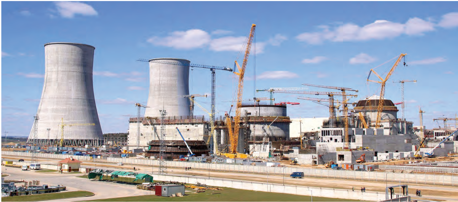
Belarusian nuclear power station construction site
