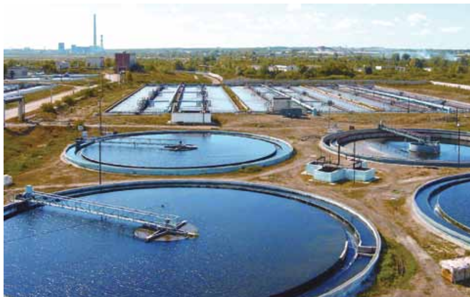
Preferential loans attracted for reconstruction of water supply facilities
