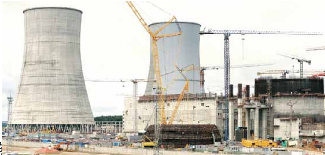
At construction site of Belarusian nuclear power station
