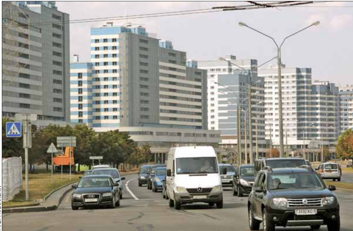
Around 4 million square metres of housing to be constructed by end of year
