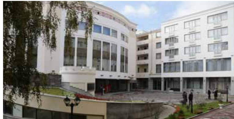
Triple-storey building of unusual architectural form perfectly suits diplomatic complex
