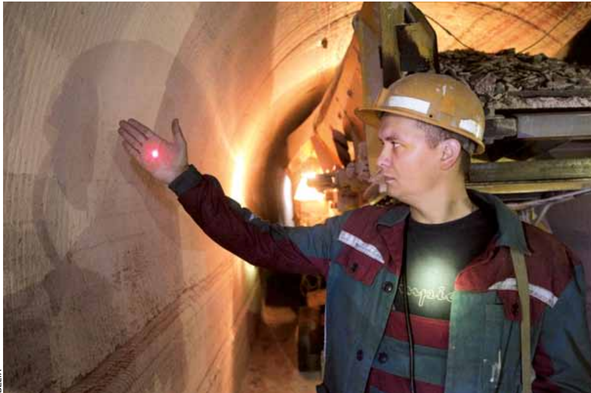
A shaft miner precisely lays tunnels with the help of a laser beam
