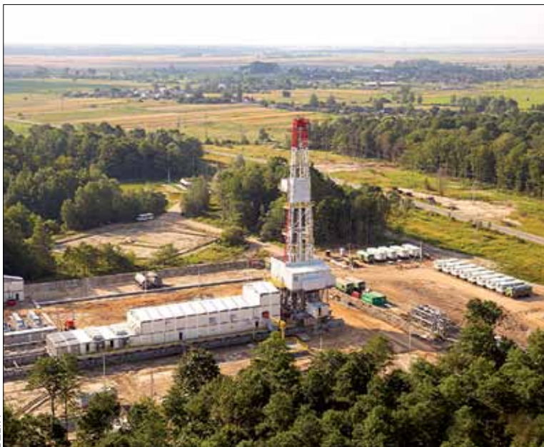
Echelon drilling rig allows to drill around ten wells
