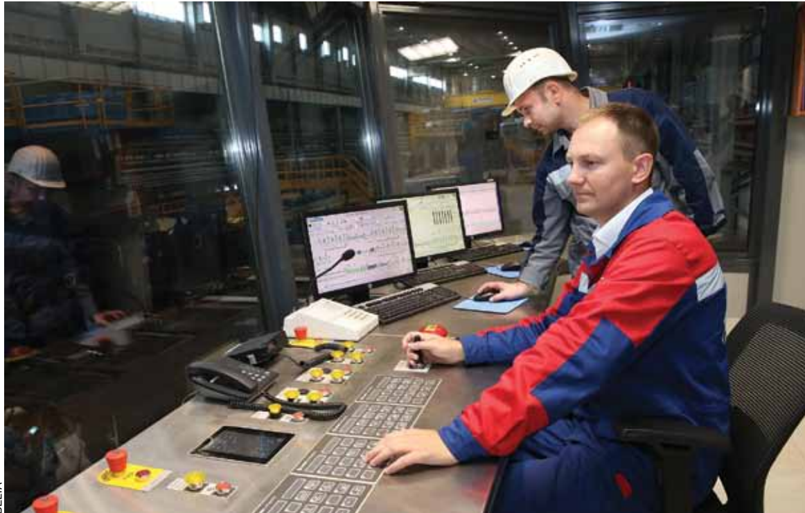
Zhlobin's BMZ new production line control centre
