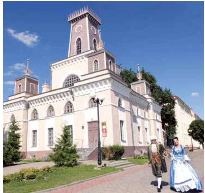
The most unusual town hall in Belarus, with towers made of wood but looking like stone
