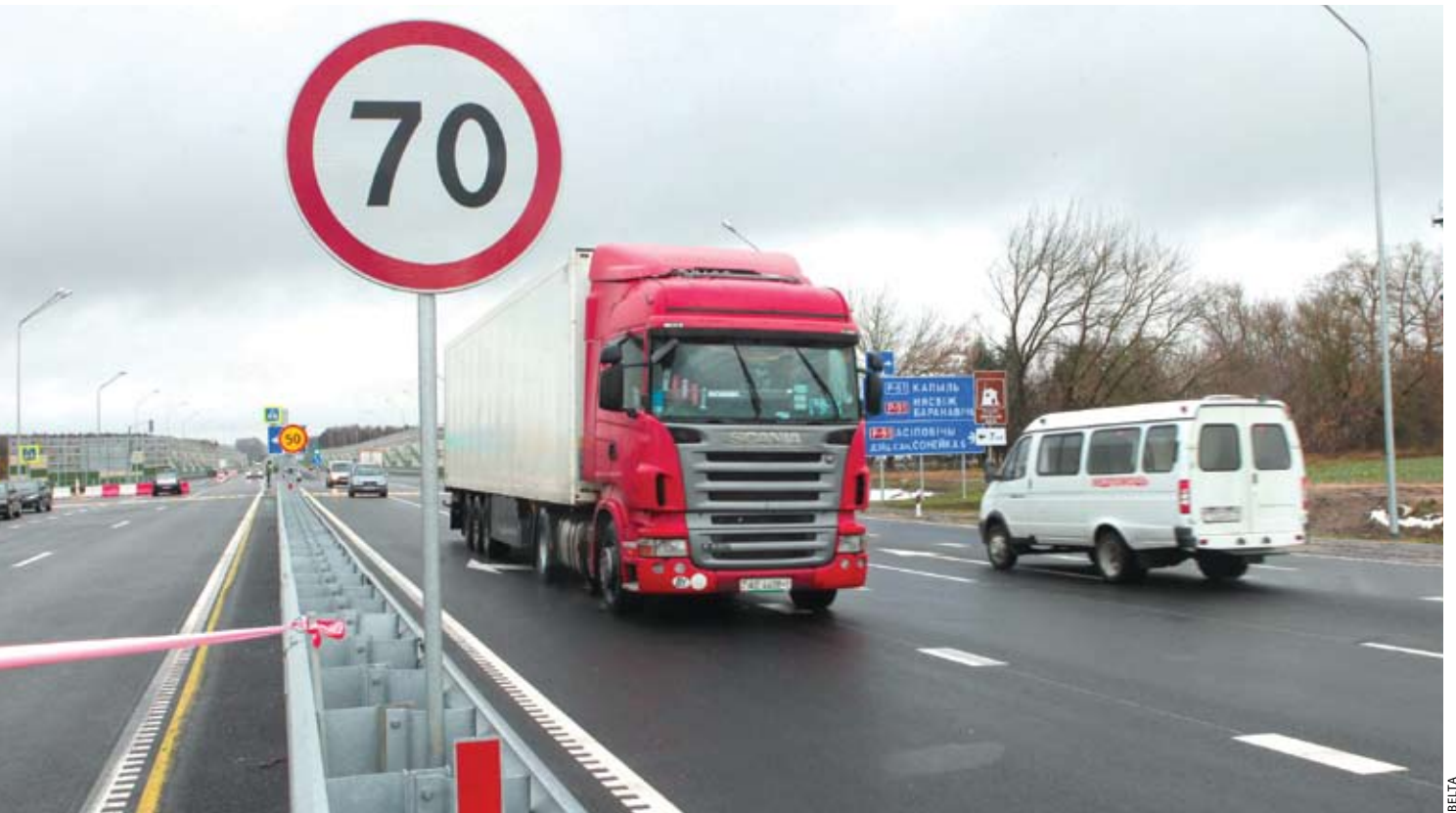
A section of Minsk-Slutsk-Mikashевичi highway after reconstruction
